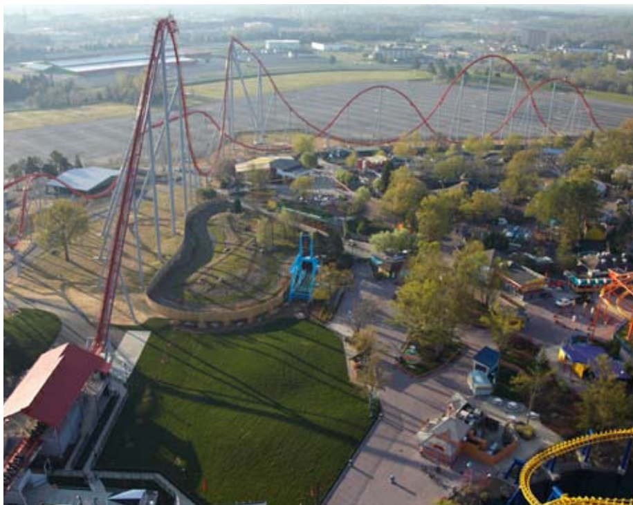
Hendrick Construction recently completed the NASCAR-themed Intimidator roller coaster at Carowinds, which opened this year as the tallest, fastest and longest roller coaster in the Southeast. The ride is named for NASCAR legend Dale Earnhardt and features a 5,316-foot track with a 232-foot peak and multiple drops and twists that reach speeds exceeding 75 mph.
