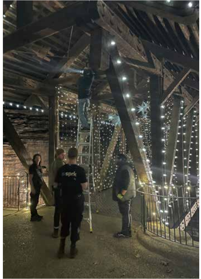
The SPRK Lighting team works on illuminating a bridge for Big Cedar Lodge. Photo courtesy of Melody Matheny
