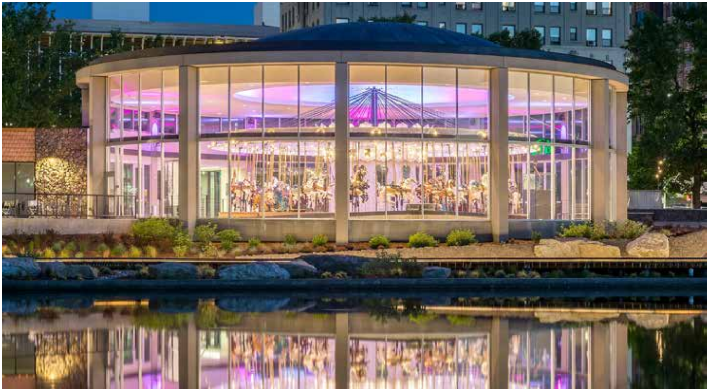
The historic Loeff Carousell in Spokane's Riverfront Park is highlighted by ETC Source Four PARs, linear LED strips, and automated wash features through an ETC Paradigm processor and a Mosaic Show Controller X controlling five distinct universes of lighting.
