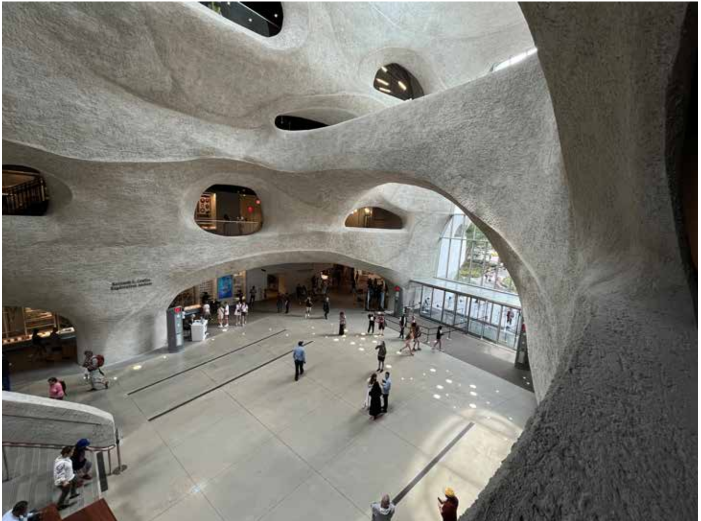
The Gilder Center is a 230,000 sq-ft addition that boasts 33 individual connections across four levels to 10 other buildings on the AMNH campus.
