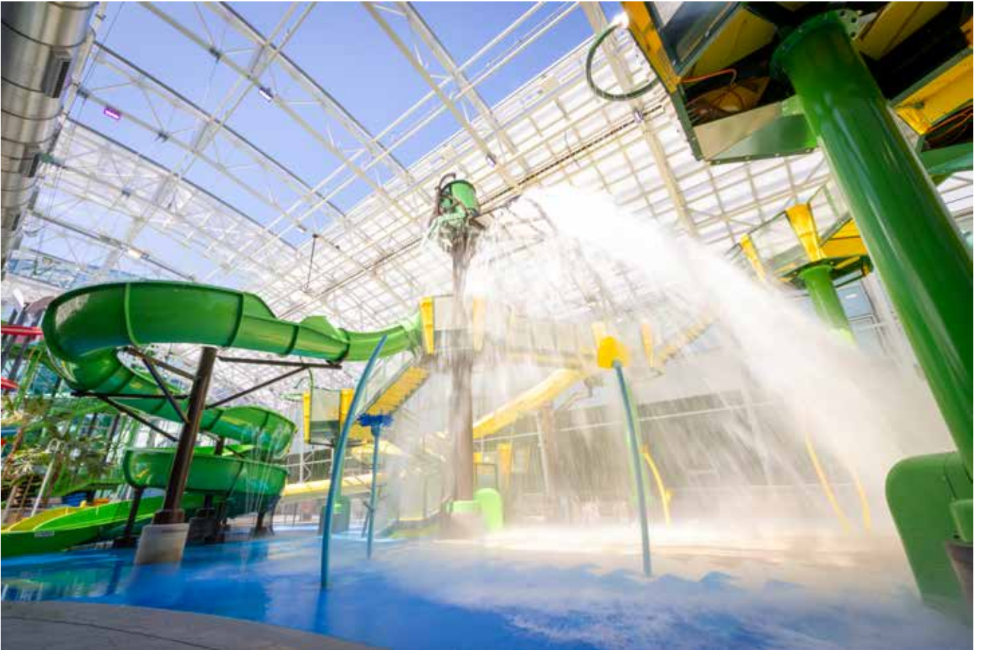
Island Waterpark at Showboat Hotel Atlantic City took advantage of the latest designs in kids' play areas, including tipping buckets that have been engineered to disperse water over a broader area.
